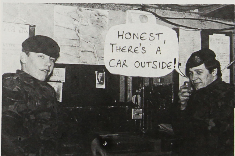
Ptes Blizard and Barrett at Clonatty Bridge (The R & R centre).
