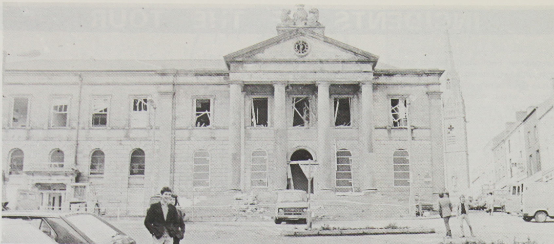
PIRA decided to celebrate the founding of the Queen's Regiment (in 1661) by blowing up Omagh Courthouse on October 14th, 1983. No-one was hurt.
