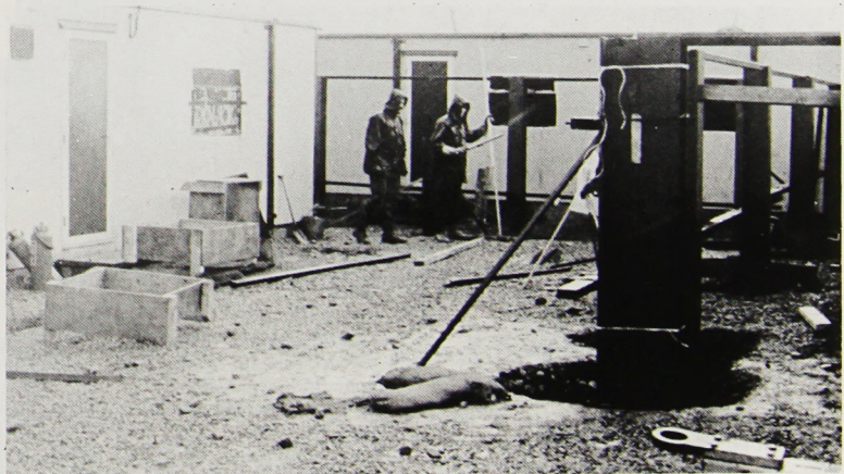
. . . requiring some modernisation.
