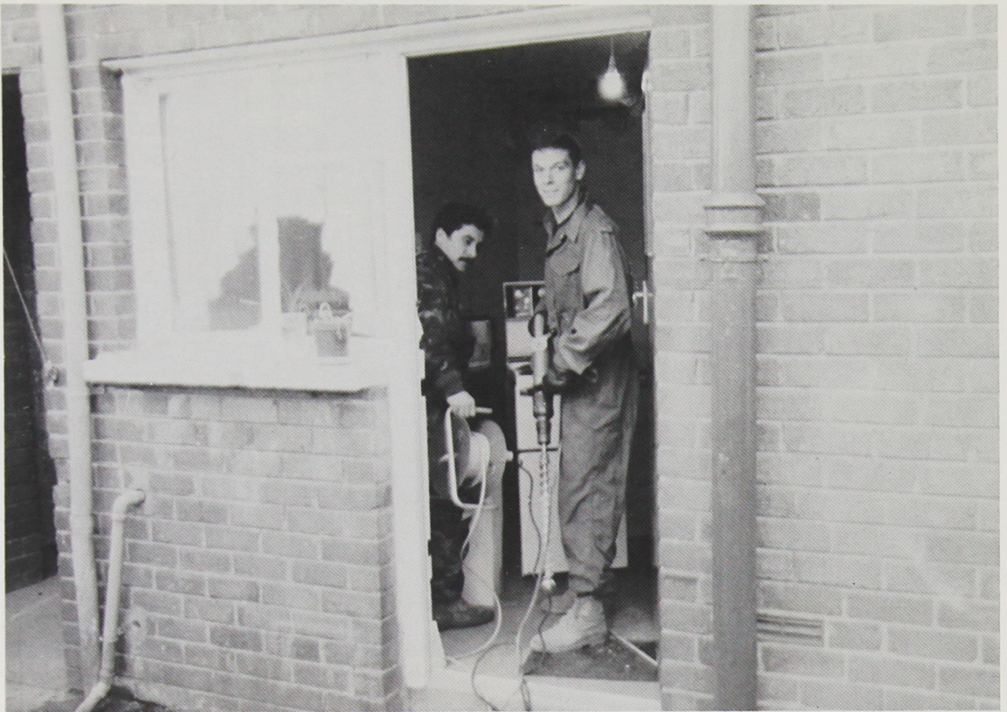
LCpl Bowart is so busy posing for the camera that he fails to notice that he is about to drill a hole in his foot. Luckily Cpl Minnis is on hand to save the day. (and the foot)
