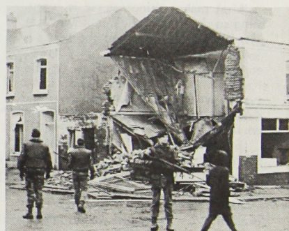
WHEN THE CHIPS ARE DOWN Major Trotman, Sgt Taylor and Pte Hooker at the scene of an explosion in a fish and chip shop in Old Park Road.
